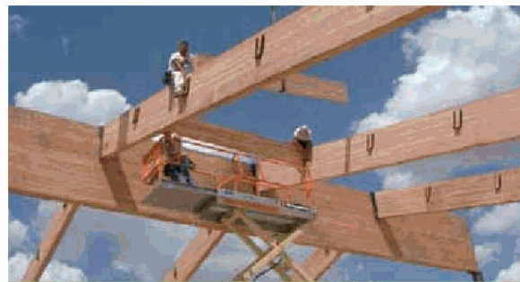
Pre-engineered glulam beams were methodically assembled on-site for the Gunter Primary School in Gunter, Texas. At nearly 60,000 square feet, wood-frame construction for the school cost just under $100/square foot. Credit: APA – The Engineered Wood Association
